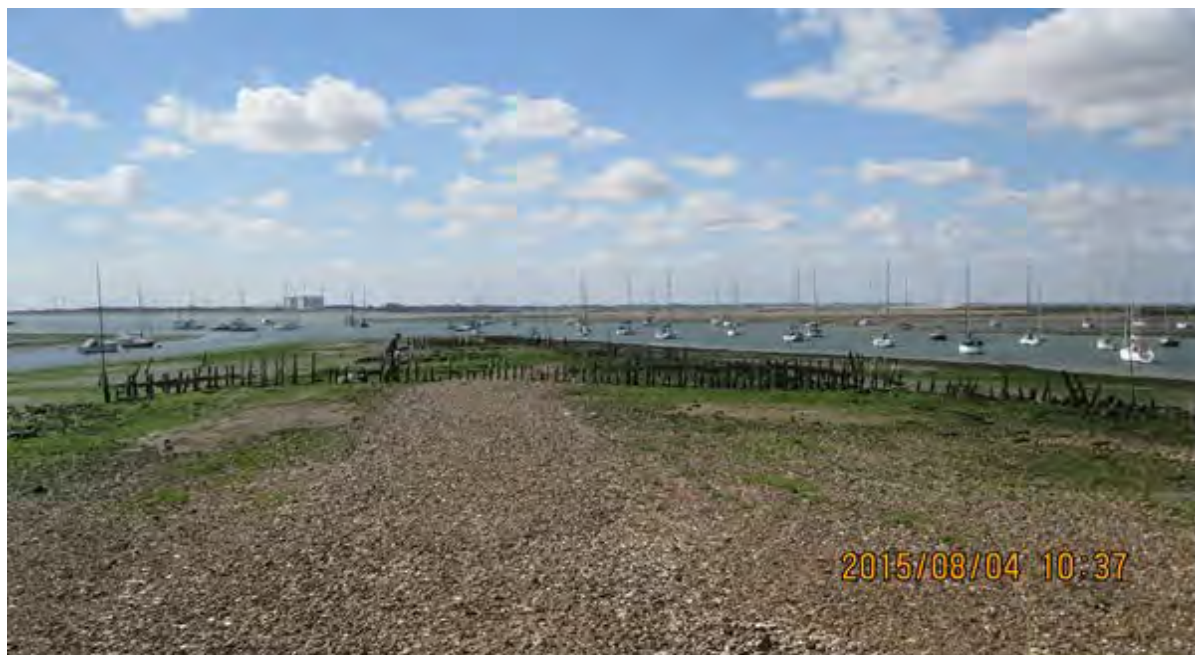
Figure 29. Packing Marsh Island - 2015 distribution of EA recharge over foreshore south of the recharge ridge formed around the oyster pits. Eroded saltmarsh platforms are situated to seaward. This is the proposed deposition site for the new recharge. The photo also shows the remains of the brushwood fencing which was erected to retain the recharge (view towards southern tip of island).
