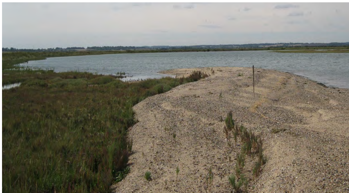
Figure 32. North-western extent of recharge reinforcing protection of the eastern tip of the sea wall, Old Hall Point. Annual sea-blite ( Suaeda maritima ) is growing through the recharge, in places.
