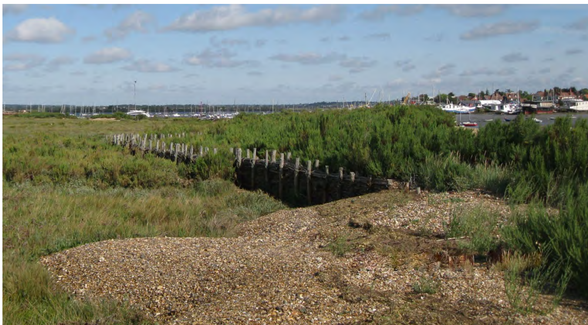
Figure 25. East shore of Cobmarsh Island where tidal forces have moved the recharge over the retaining fence onto the marsh. Shrubby sea-blite ( Suaeda vera ) has colonised and stabilised the recharge ridge both inside and outside the fence (view north). The similar grading curve of the imported material allows it to be reworked by wave action and storm events in the same way as the naturally occurring material (see Figure 24 above).
